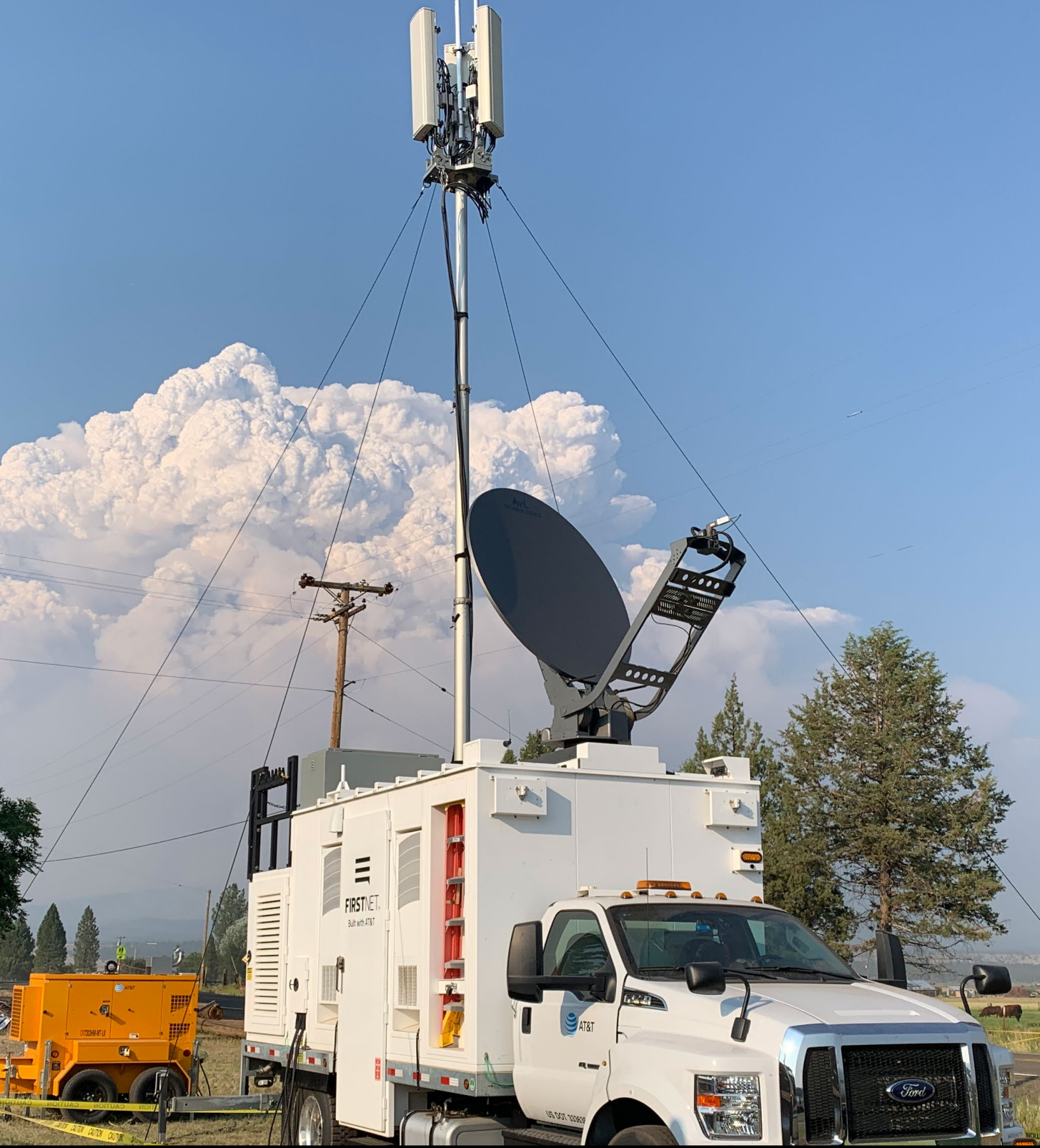
A FirstNet SatCOLT deployed to the Bootleg Fire in Oregon. These mobile cell sites link to FirstNet via satellite, do not rely on commercial power availability, and provide similar capabilities and connectivity as a cell tower.
